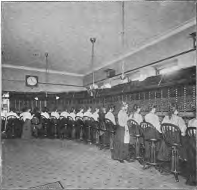
Switchboard in a Central Telephone Office
